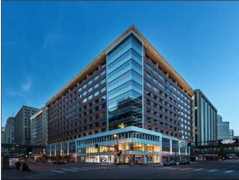
**Figure 1. Striking glass curtain wall extending 12 stories and expanded window lines on street level that showcase the entrance lobby**
