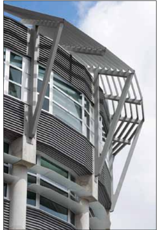
Figure 1 Windows on top floor feature sunshading devices
