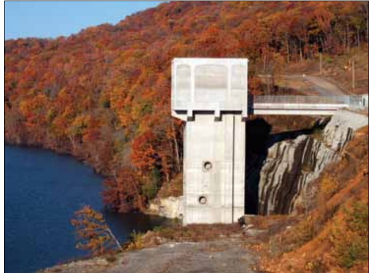
Figure 1 The concrete intake tower at Lake Fort Smith State Park.
