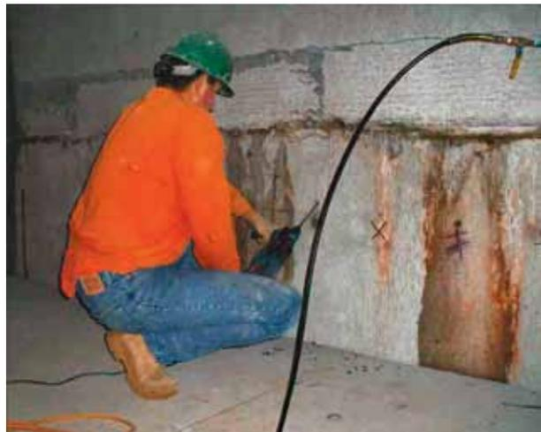
**Figure 3** Drilling continues along the construction joint.
