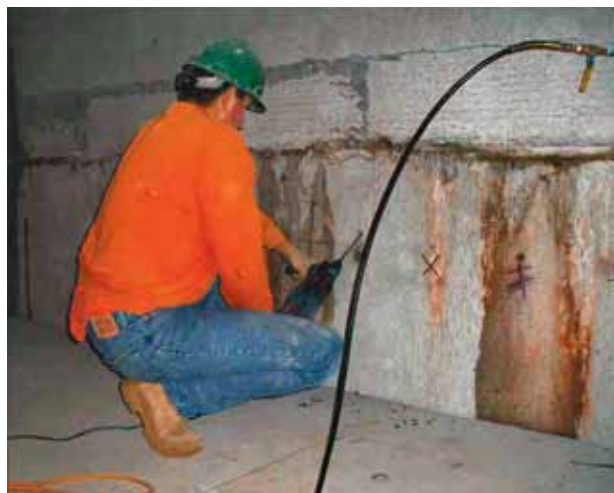
Figure 3 Drilling continues along the construction joint.
