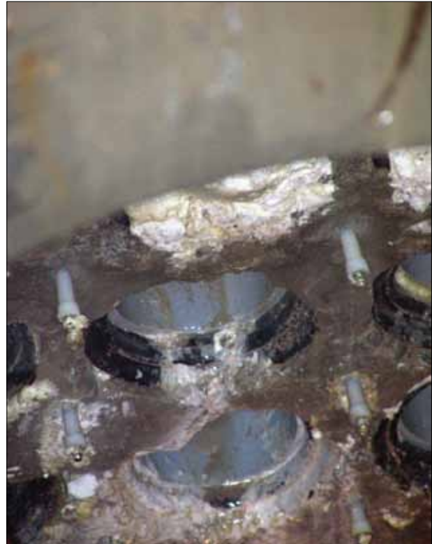
Figure 3 Close-up of the injection site.
