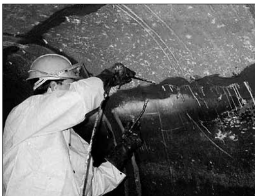
Grout installation in a manhole.
