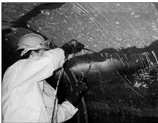
Grout installation in a manhole.
