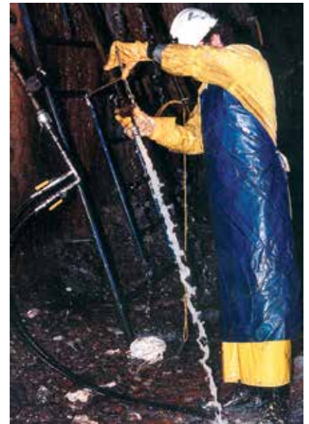
Azo-Grout™ being used in a gypsum mine with a multi-ratio pump.
