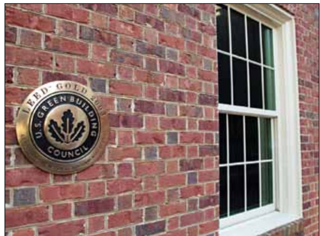
Figure 2 Completed in 2003, Hipp Hall at Furman University in Greenville, SC., achieved a “Gold” LEED rating, the first building in the state to receive this certification.
